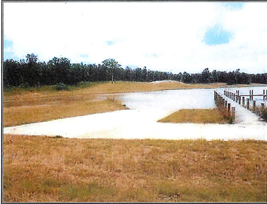
Viewing boat ramp in the northeastern portion of lake
