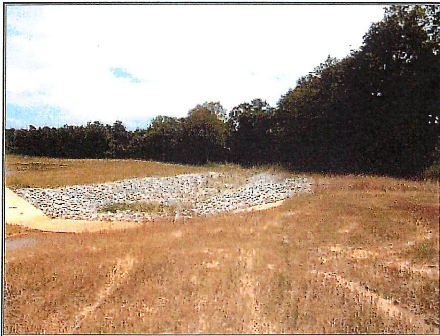
Viewing spillway in the northwestern area of lake
