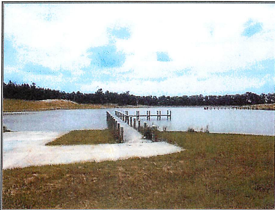
Viewing boat ramp/pier in the northeastern portion of lake
